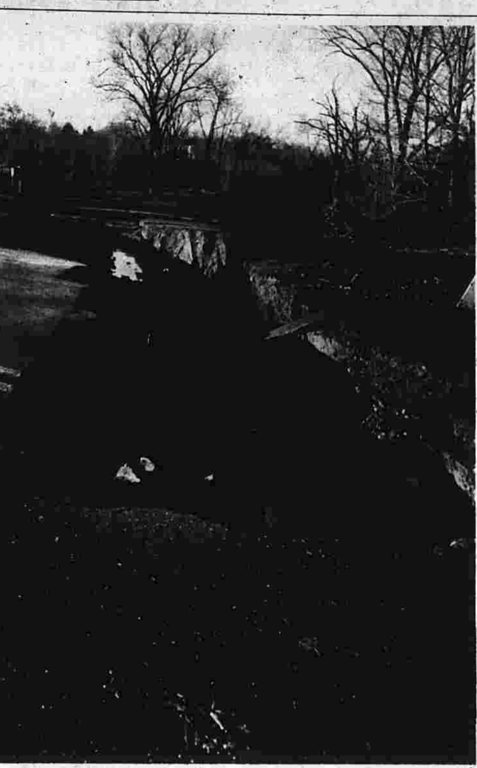
Rains Cause Cave-In at Union St. This is Union St. where last night's heavy rains caused the road to cave in. The collapsed area almost blocks all of Union St., leaving only a narrow place to pass.
